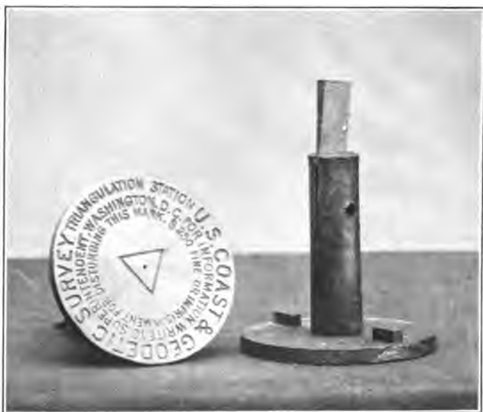
FIG. 2.—STANDARD TRIANGULATION STATION MARK.
